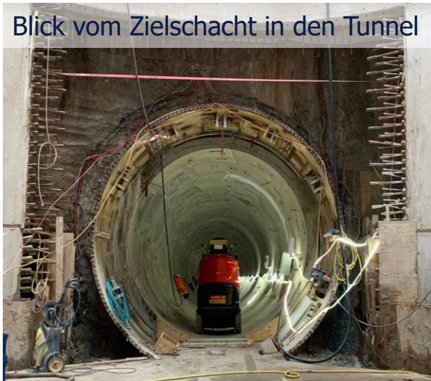
Blick in den Tunnel
