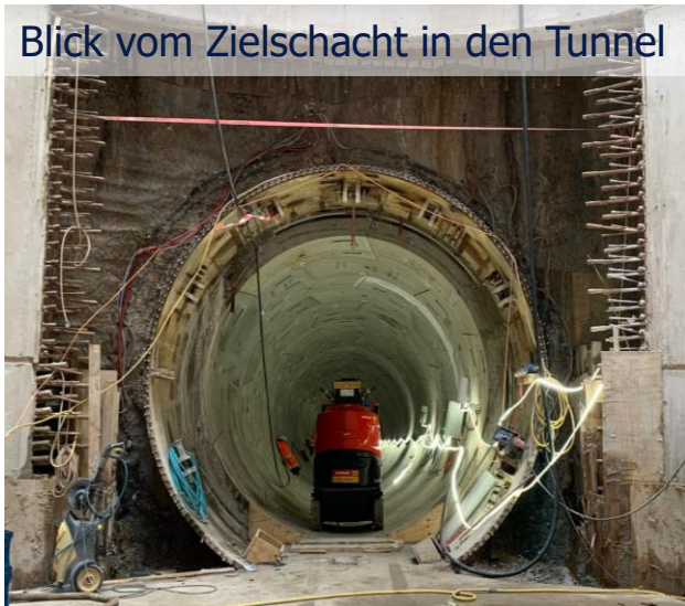
Blick in den Tunnel
